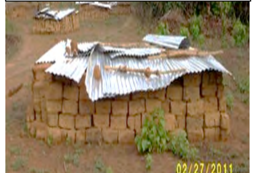
Mud Building Blocks for Kondesu Clinic
